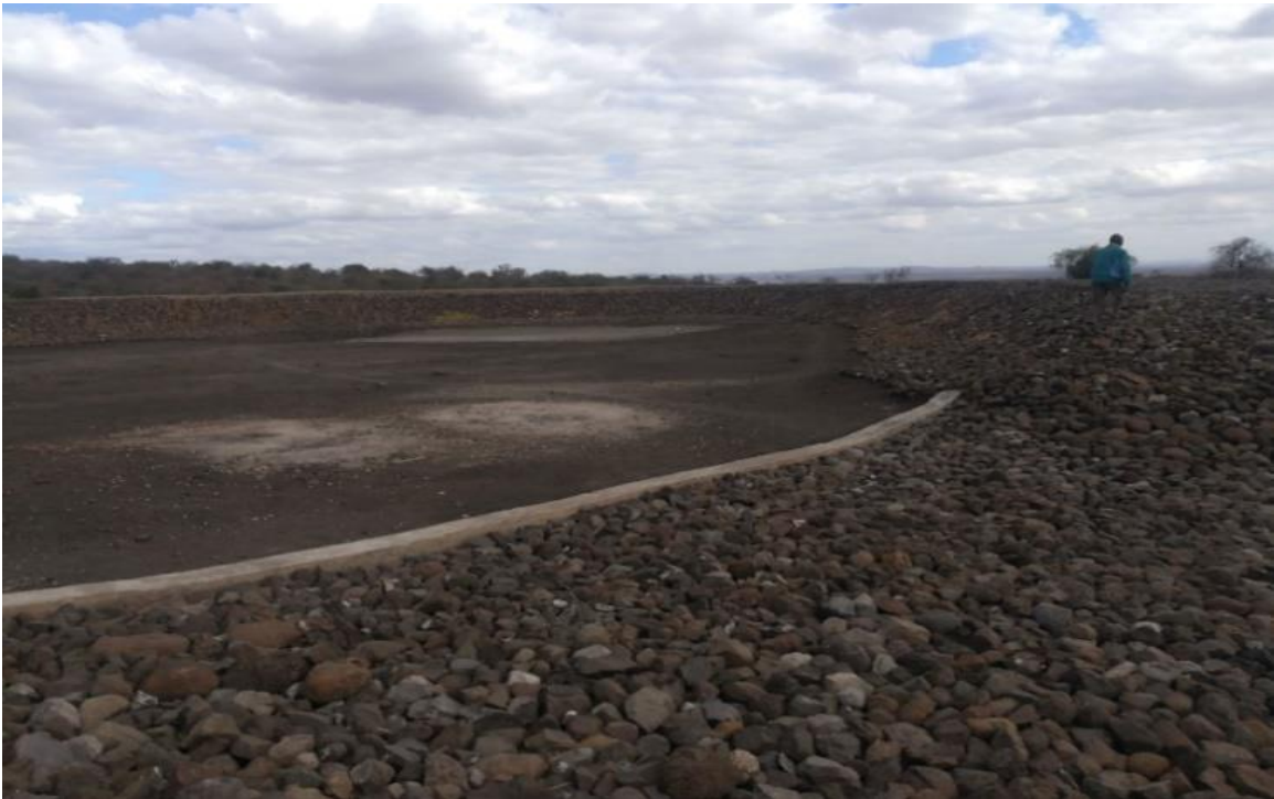
Picture 6: Constructed charco dam in Mbuyuni village in Monduli.
