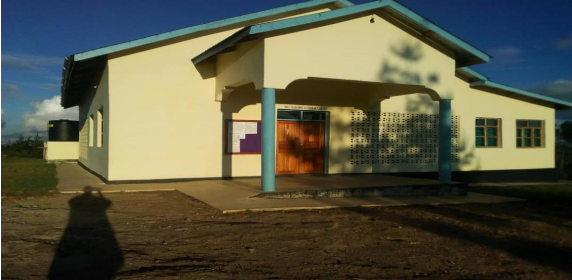
Picture 5: Health facility constructed at in Lupombwe, Makete.
