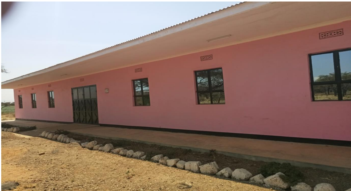
Picture 2: Girls' hostel constructed at Qangdend Secondary School, Karatu.
