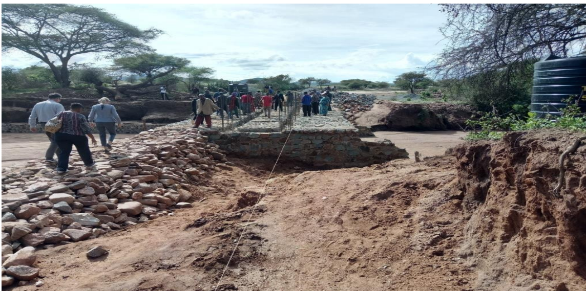
Laja bridge in Karatu still under construction through public works program.
