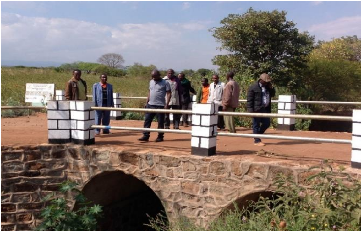
Picture 7: Bridge rehabilitated at Gyekrum-Lambo road in Karatu District.
