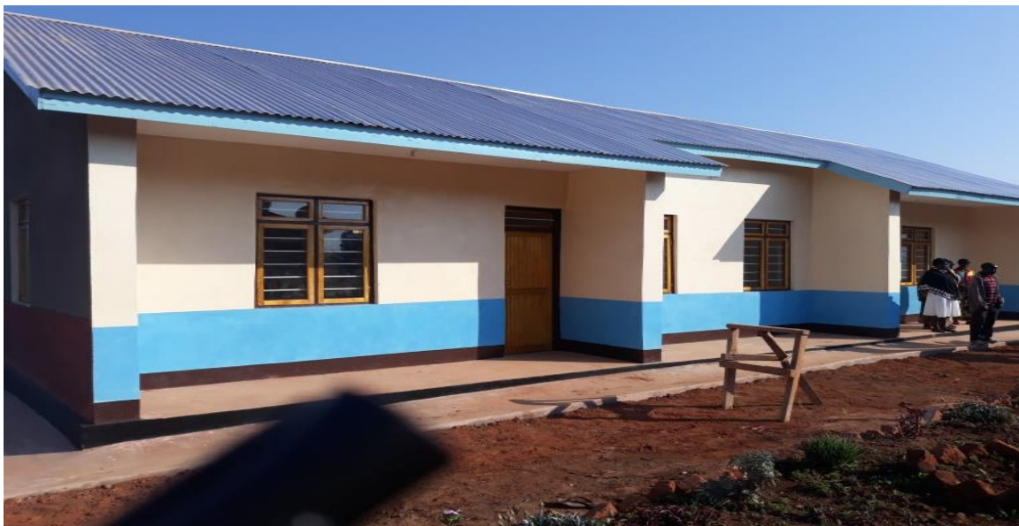
Picture 4: Nurses' two-in-one house constructed at Ilininda Village, Ludewa.
